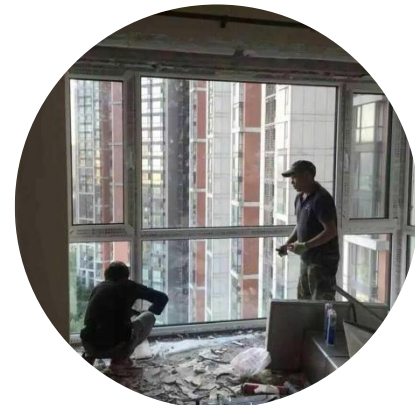
Windows and doors installation
