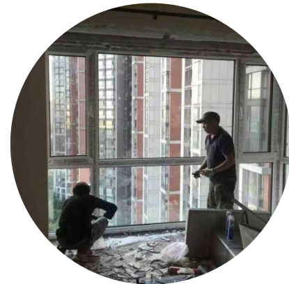
Windows and doors installation
